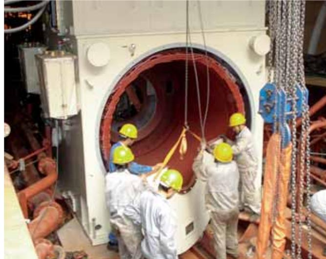
Installation of a shaft generator
